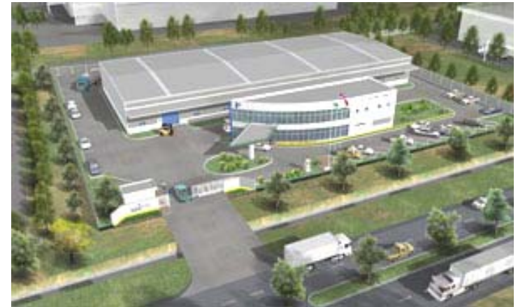
Ota Techno Park in Amata Nakorn Industrial Estate, Thailand (less than 1 hour from Bangkok)
